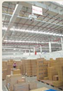
Skylight on the plant roof
